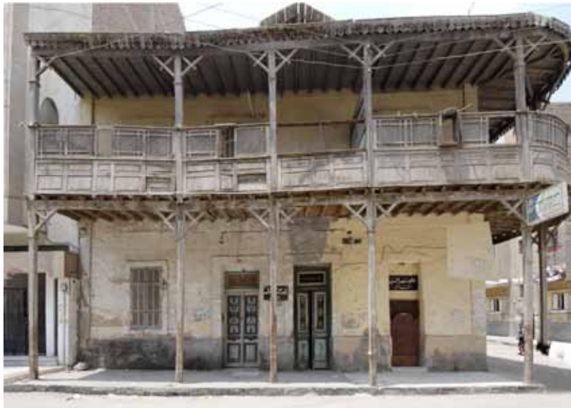
Housing in the Arab quarter, Ismaïlia, Egypt, c. 1885 (source: © Arnaud du Boistesselin, 2008). The verandah-solution of the façade, characteristic of 19th century "tropical" European architecture, was enforced by building regulations applied in the cities along the Suez canal until the 1920s.
