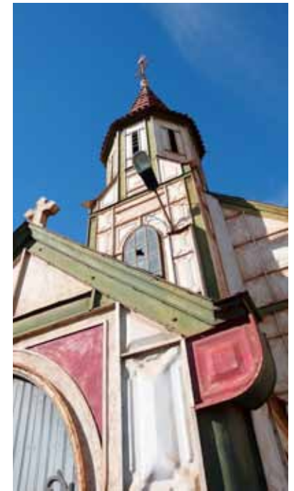
Prefabricated metal church, Boma, DR Congo, 1889. Design: Forges d'Aiseau (source: © Johan Lagae, 2009).
