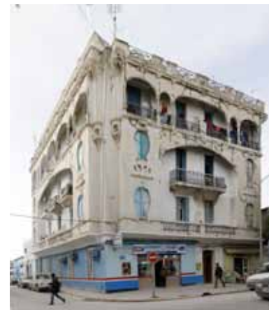
Azerm Building, Tunis, 1905-1906 (source © Arnaud du Boistesselin, 2010).
