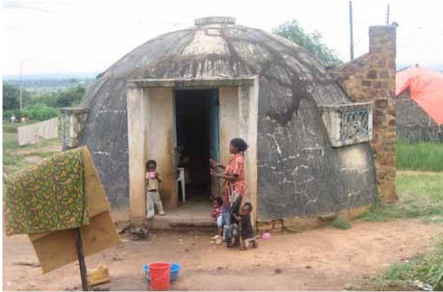
"Balloon House" in the quartier Tshamilemba, Lubumbashi, DR Congo. Based on an invention of the American architect Wallace Neff, this concrete housing type arrived in Lubumbashi in the early 1950s after having been seen applied on a massive scale in Dakar, Senegal (source: © Johan Lagae, 2006).
